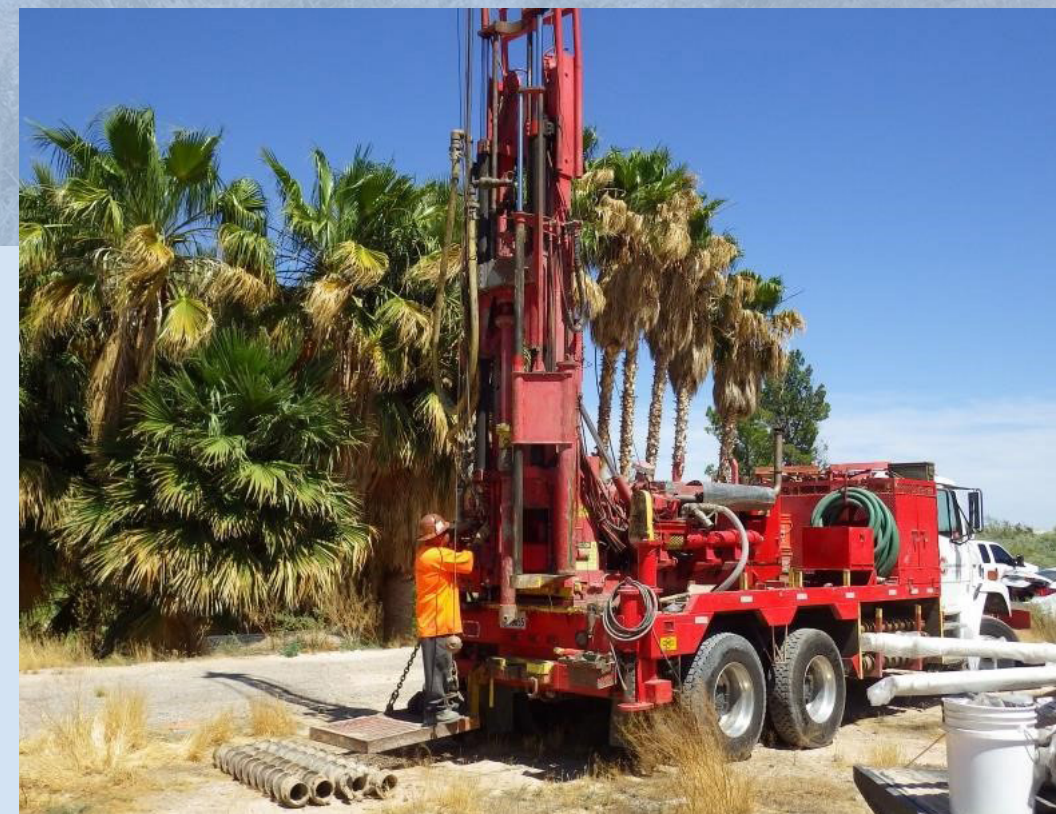
Installation of groundwater monitoring wells
