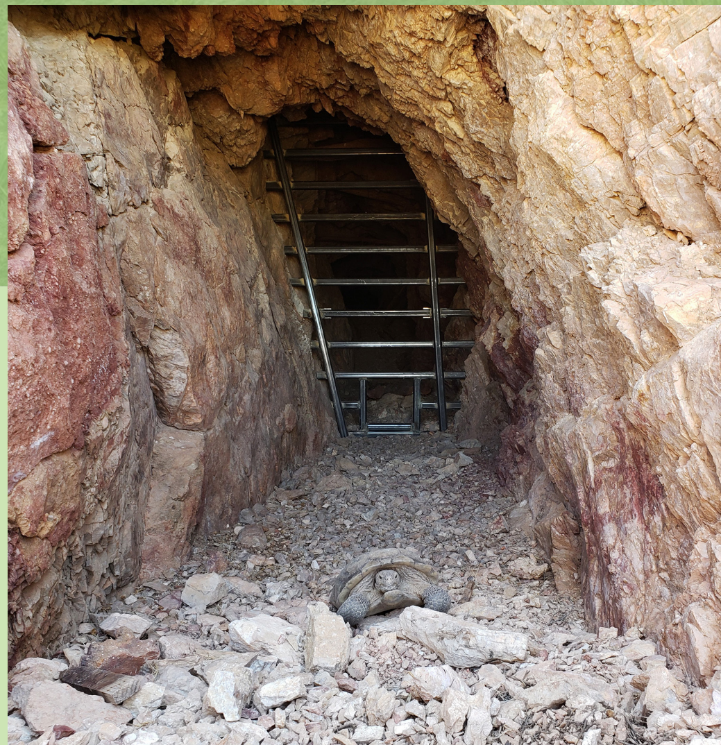
A wild desert tortoise exiting an AML with a recently installed wildlife compatible closure featuring a custom tortoise entryway at Gold Butte National Monument.
