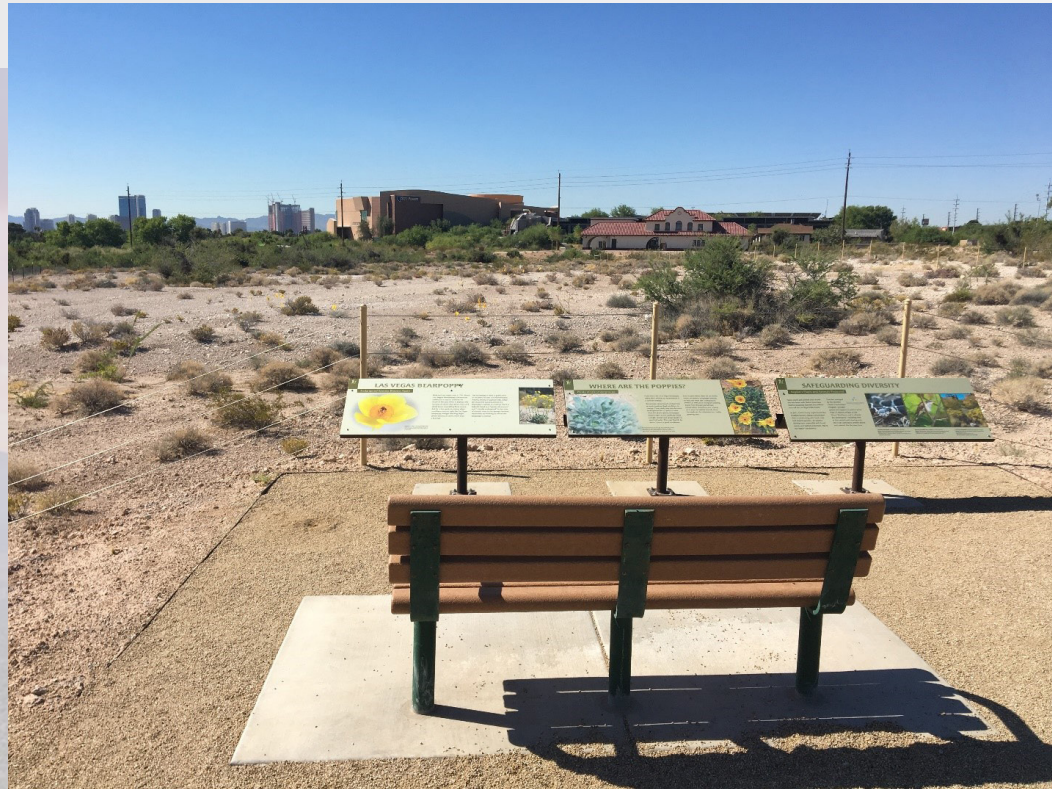
Bearpoppy viewing ramada constructed at the Springs Preserve
