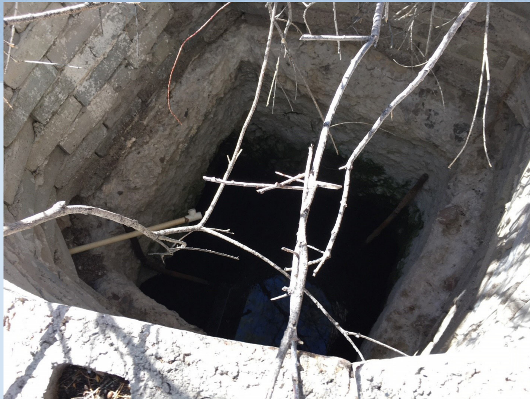
Hazardous condition at Summit Spring, pre-restoration
