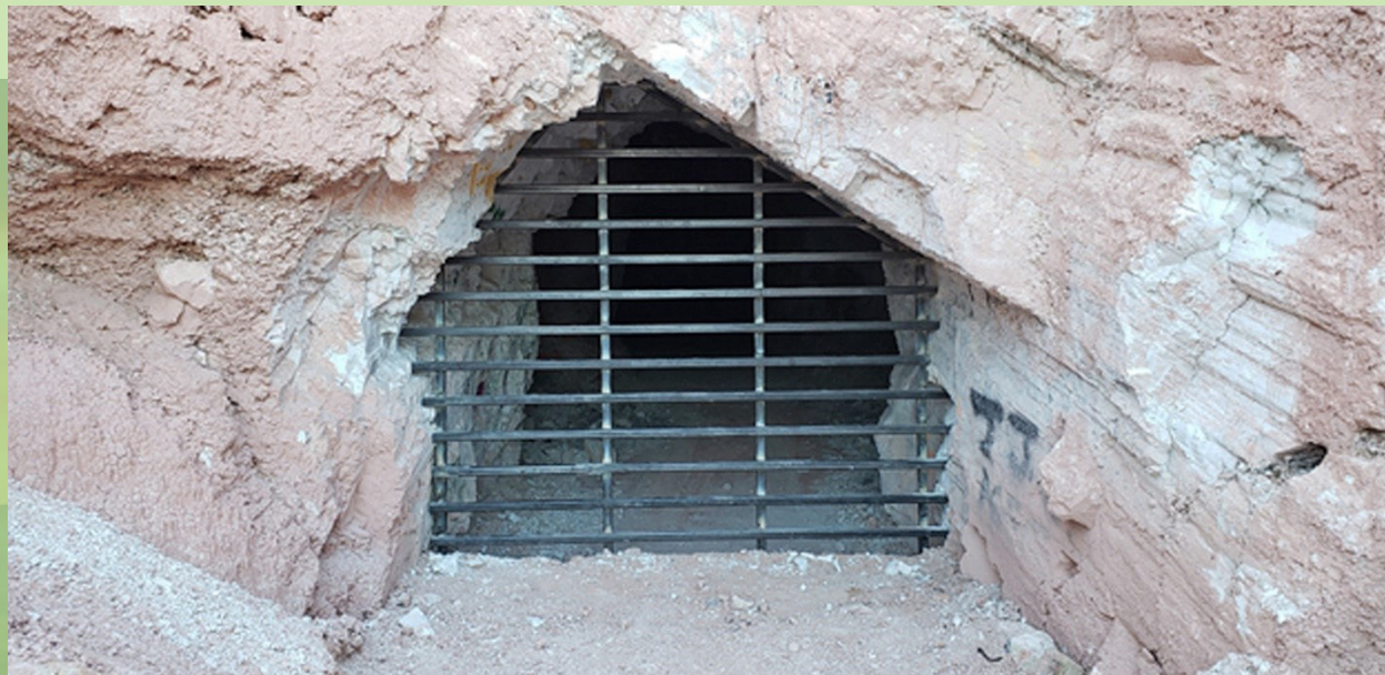
A wildlife compatible closure installed at an AML in Valley of Fire State Park.
